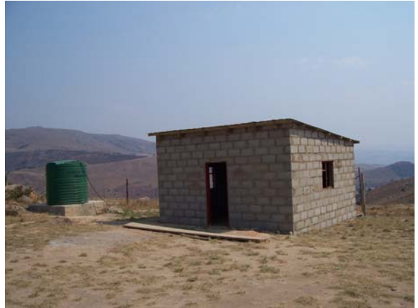
New Kitchen Being Built at El Shaddai School
