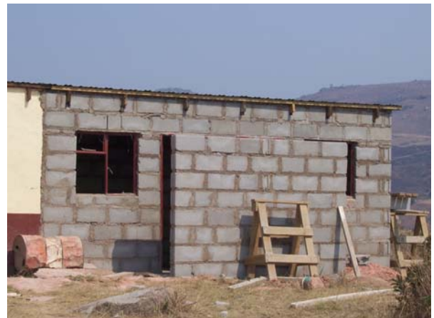
New Bathroom with Flush Toilets Being Built
